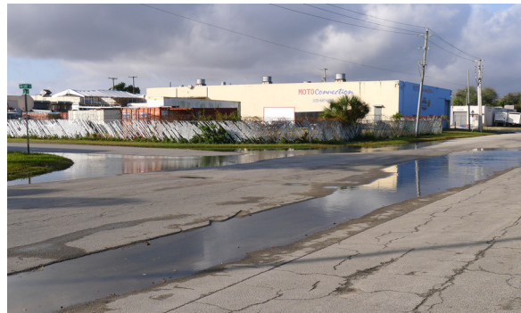
Fig. A.12: Deteriorating pavement and poor drainage are typical of streets in the Opa-locka commerce area. (NW 147th Street)
